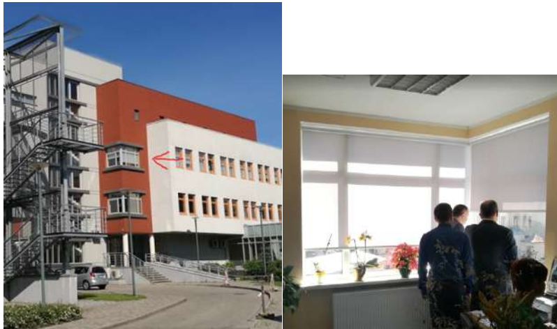
Figure 35 - UC3 D2: (Left) Laboratory building with laboratory on 3 rd floor (see red arrow). (Right) Laboratory room from inside
