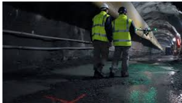
Figure 9 UC1 – Drone during inspection work in tunnels
