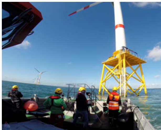
Figure 52: Inspection of offshore turbines structures
